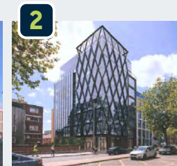
2 The Greenside Building 10 storeys
